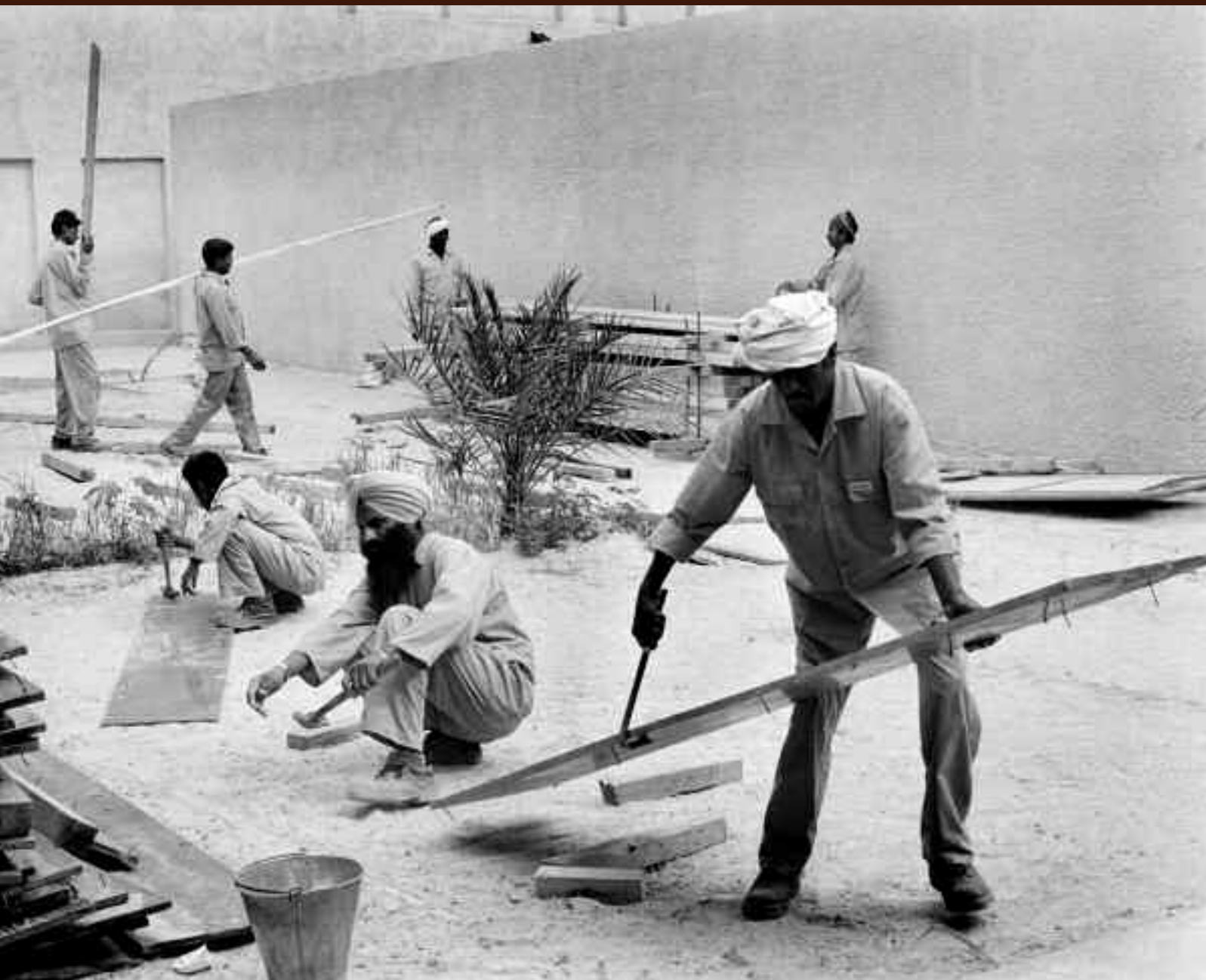
Workers renovate the Arab quarter of Bastakia.
